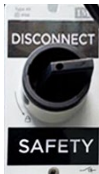
Figure 8c. Example of Strand-Mount Antenna EPO Switch
