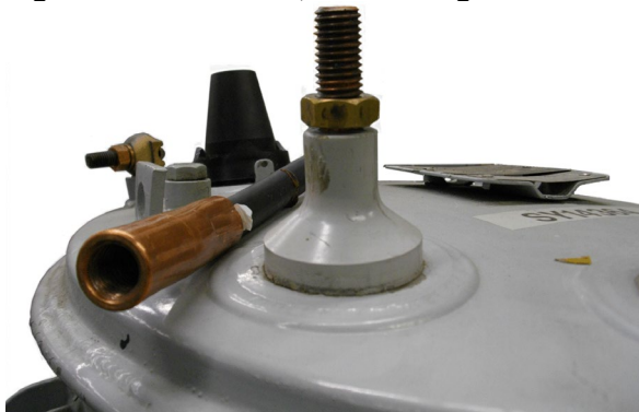
Figure 6.3a Threaded, Low-Voltage Terminal Stud
