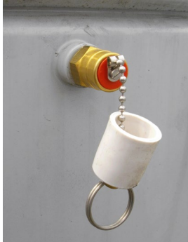
Figure 6.8.1 Pressure Relief Valve
