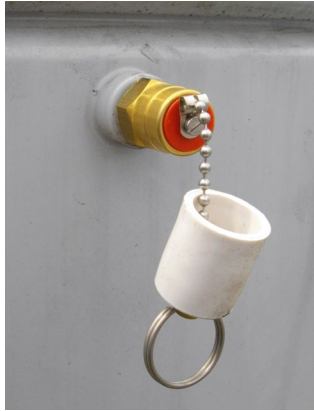
Figure 6.8. Pressure Relief Valve
