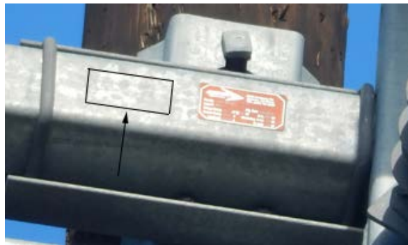
Figure 4h. Installing Location: To the Left of Nameplate
