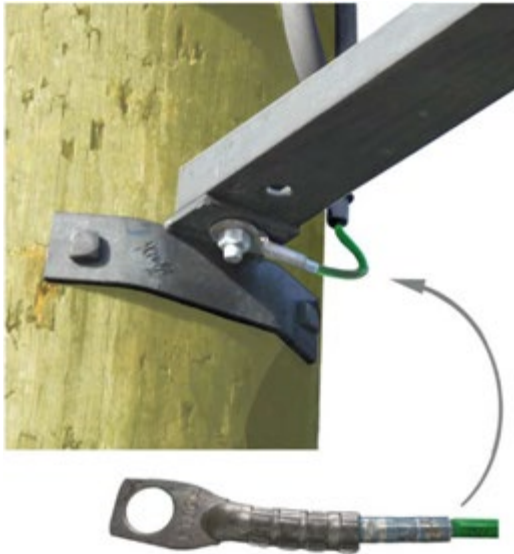
Figure 4c. Routing Ground Wire
